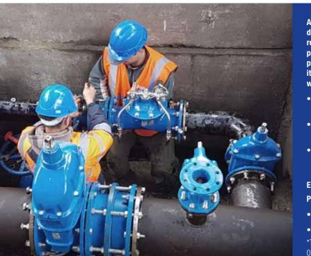
After installation of 235 valves, overall water distribution in the supply area has been reduced by seven percent compared with the past year. The risks of water hammer and pipe bursts are minimised, and the electricity consumption and the amount of pumped water is reduced;
